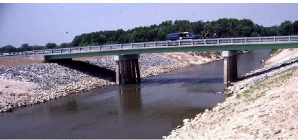
Incision undermined bridges (lots of new bridges here!)
