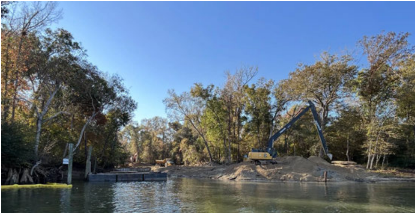
Barging out excavated sand from Spiders Cut, Nov 2025
